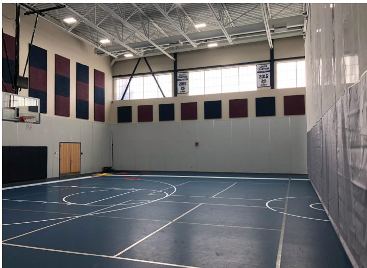
New LED lighting in the Sizer School's gym.
