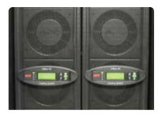
By placing the cooling directly where it is needed (washing the face of the servers), and recirculating the discharge heat before it mixes with the remaining space, the Markley Group gets optimal efficiencies.
